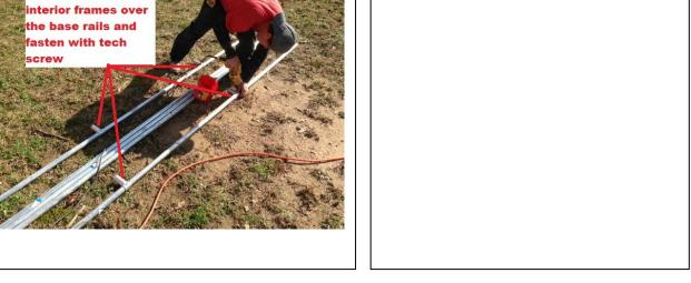
Both the front and rear end base rail must be 144" long before installing them into the 3-way corners, it can be one joint 10'6" long factory joint, if the factory tubing has a small swaged end and they usually do then add a 21 1/2" pc onto the swaged end full joint in which case you will not need to use the supplied splicer's. The measurement of the added pc will be longer if using un-swaged or tubing other that 10'6" factory length tubes.
