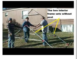
Then push each of the three purlins through the peak and two side eve connectors. Position the frame sets on the marks on the purlin then secure with tech screw.
